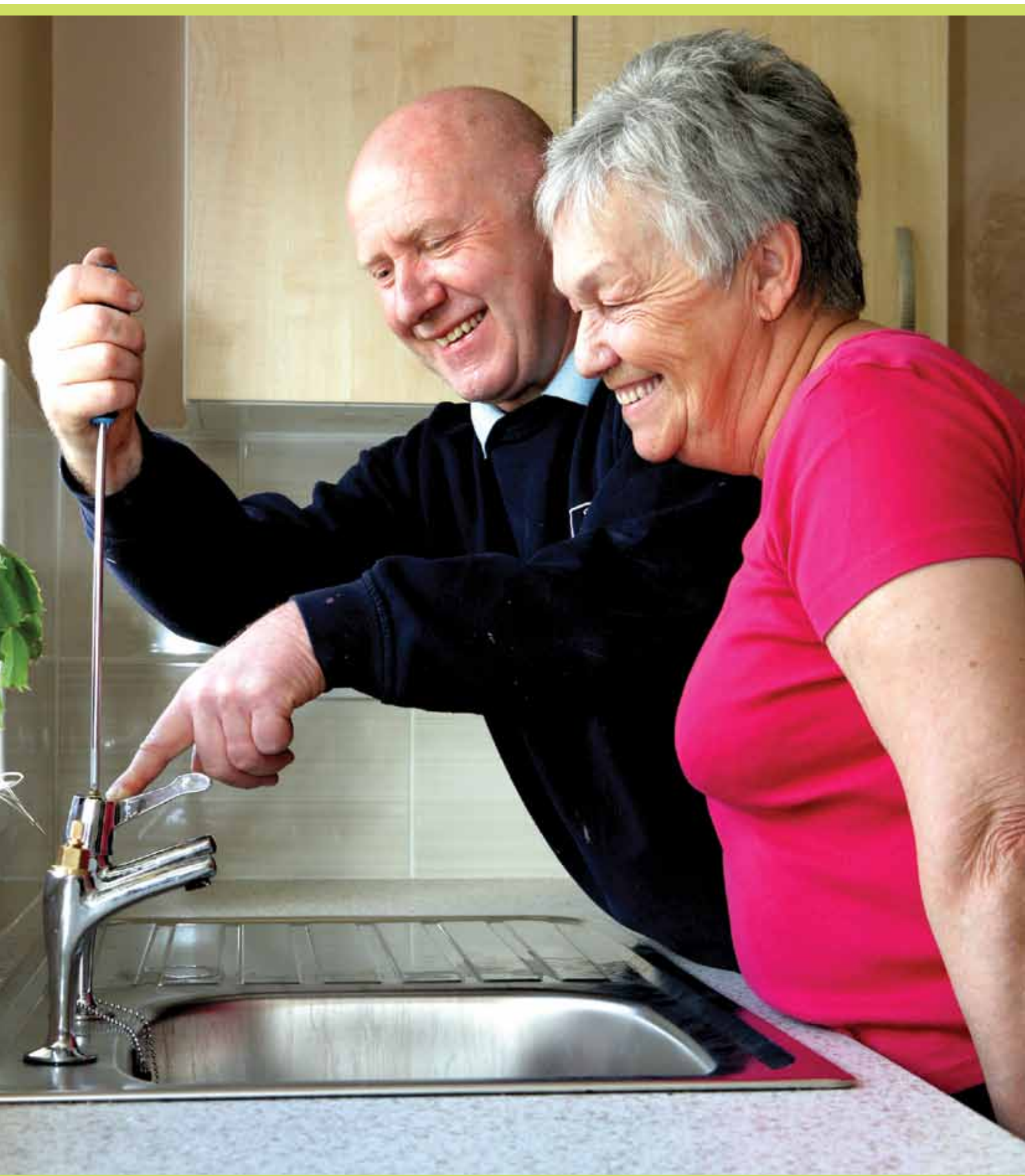
• A St. Legers Homes of Doncaster plumber, Steve Oakley, pictured with tenant Susan Bailey, performing a repair in her home
