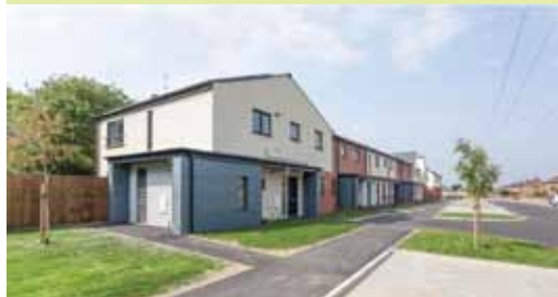
• New build homes to be managed by Colchester Borough Homes (photo © Rose Builders Ltd.)
