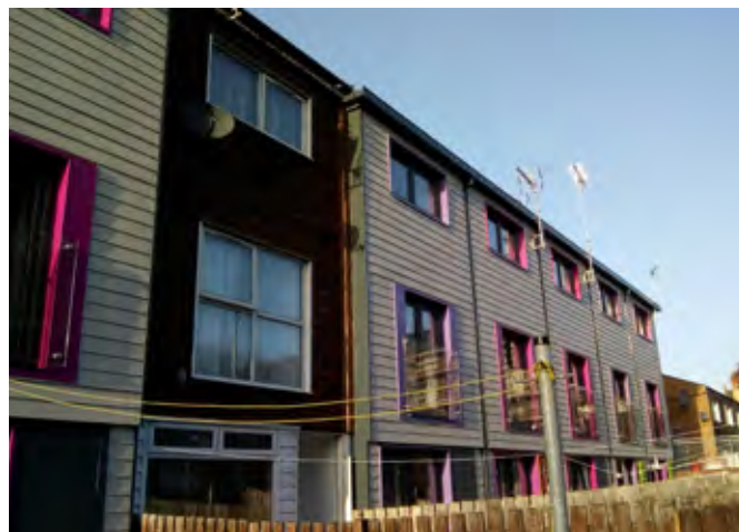
NCH's pilot scheme terrace retrofitted to 2050 net zero-carbon targets – the privately owned home pictured here opted out of the retrofit
